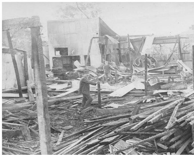
Source: State Library of SA, Fire Damage at Buttery Brothers, PRG 280/1/33/121
